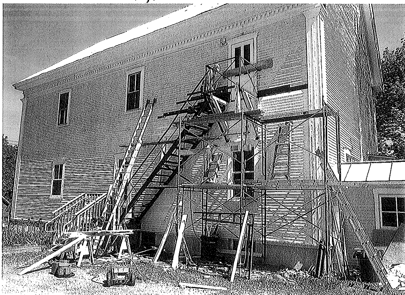
CLAPBOARD REPLACEMENT ON SOUTH SIDE NEARING COMPLETION
