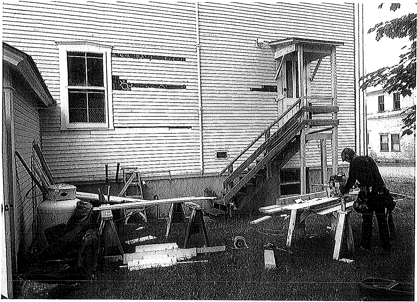
SOME CLAPBOARDS ON EAST SIDE REPLACED, MORE REMOVED
