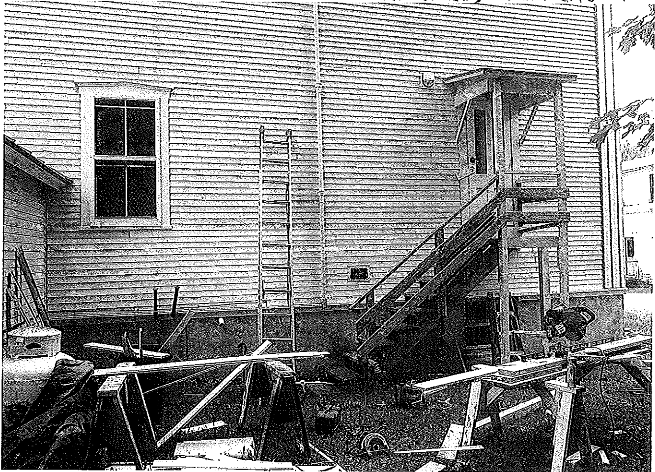
CLAPBOARDS & ROT REMOVAL NEARING COMPLETION
